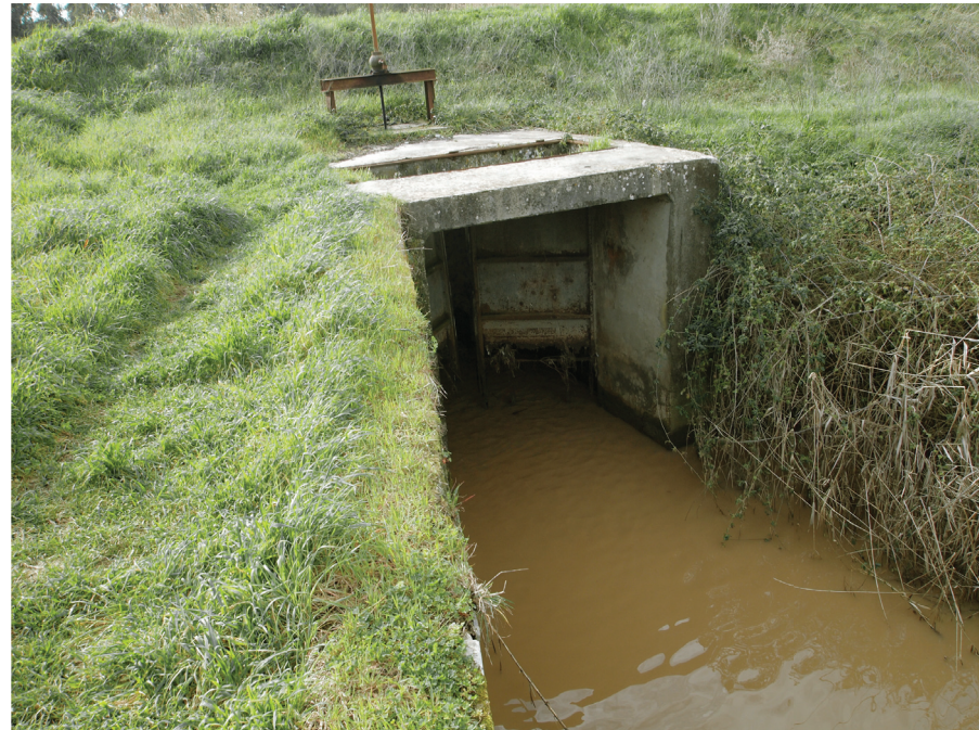
Figure 2 Hydraulic connection between Moscarello Channel and Colmata river
